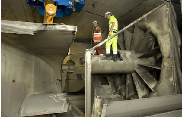
Demontage alter Abluftventilator
